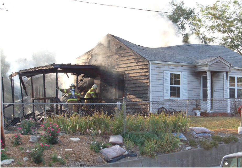
Firefighters inspect the damage after putting out a fire Sept. 4 at the 700 block of N. Osteopathy St. The property damage is estimated at $80,000. Emily Battmer/Index
