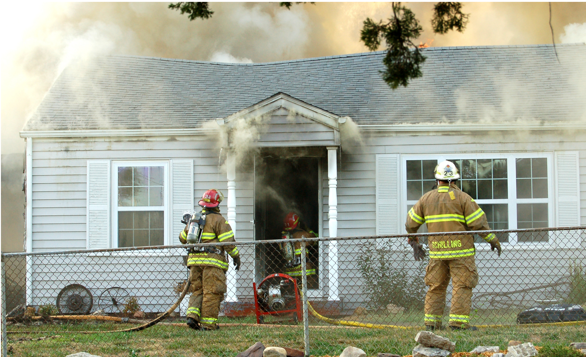
Firefighters attempt to put out a fire that damaged a house Sept. 4 at the 700 block of N. Osteopathy St. Sept. 4. No one was in the building at the time of the fire. Emily Battmer/Index
